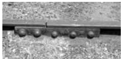
75lb on the left, and 80lb on the right. Opposite side of the other photo, as markings on the plates on this side give it away
