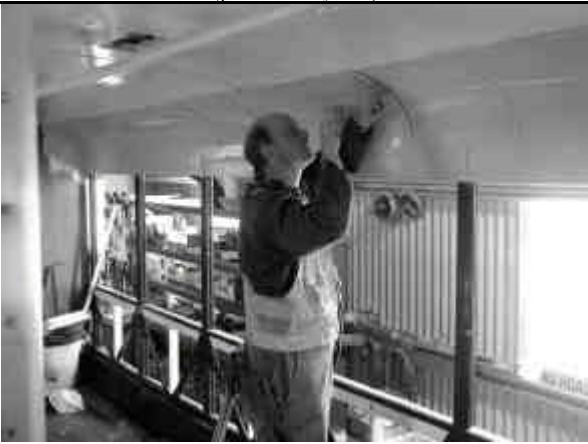
Attaching strengthening ribs to aluminium panels.
