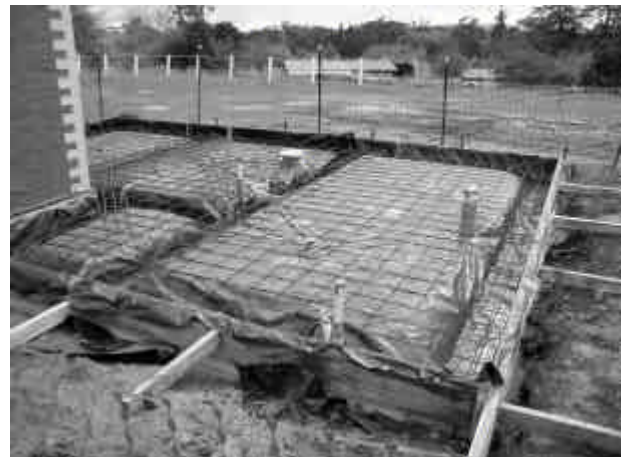
Foundations being laid. (photo B.Fell)
