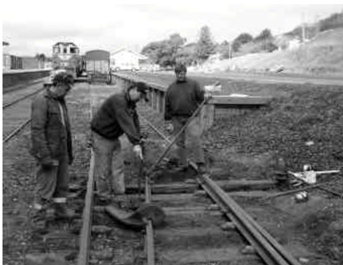
Straightening a bent point blade with a buda jack, Daylesford yard # 3 road.
