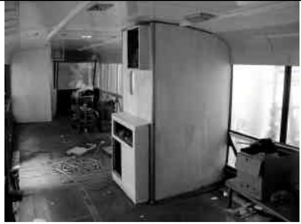
Toilet cubicle and driver's cab wall after painting with sealer / undercoat.
