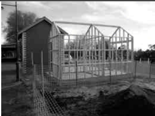
Frame for storage & disabled sections being erected. (photo B.Fell)
