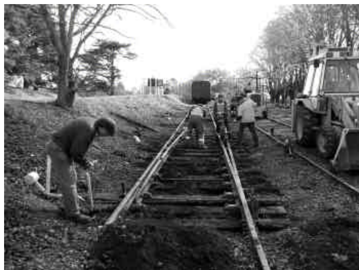
3 ways of packing sleepers - by hand, by using a petrol wacker, and the tamping machine (in the background).
