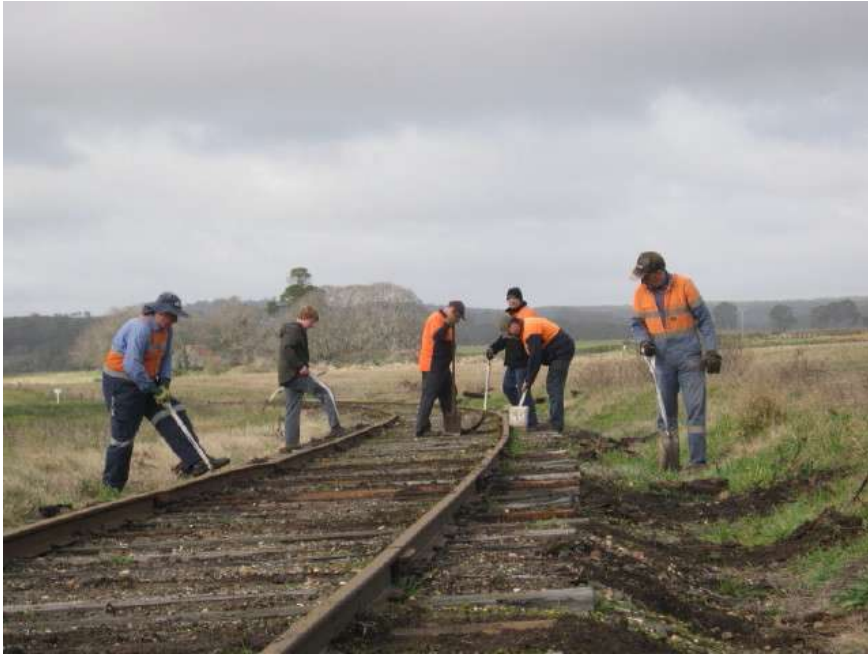
Volunteers boxing in the track after contractors had replaced sleepers.
