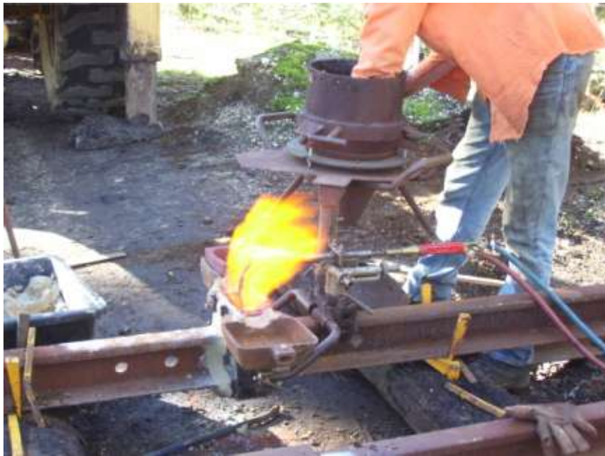
Heating up rail heads while preparing the crucible.
