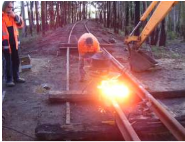
8 May 2010: Weld in progress with steel flowing out of crucible. Photo: Donald Sharp
