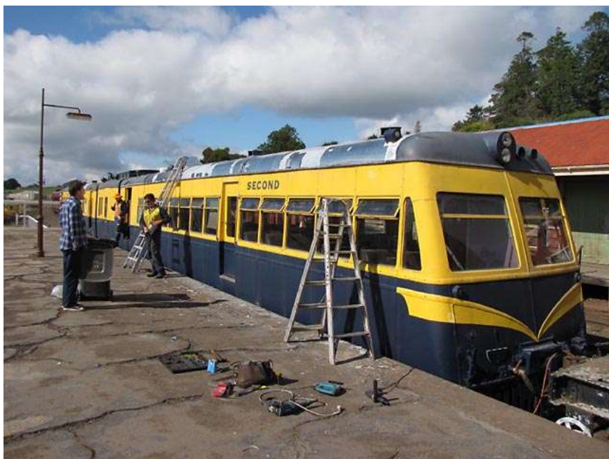
Roof work on 91RM continues, April 2010.
